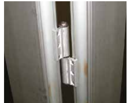
Picture 2: Mid-hinge (Opened position)
